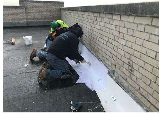
Figure 12: set fleece reinforcement into fresh PMMA resin.
