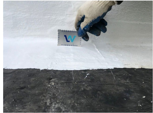
Figure 16: verify 2 nd PMMA resin coat is minimum wet 45mils thick.
