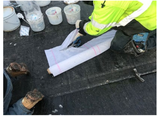
Figure 4: Pre-cut and dry fit reinforcing fleece.
