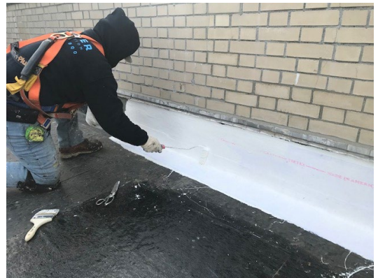
Figure 14: saturate fleece reinforcement with 2 nd PMMA coat.
