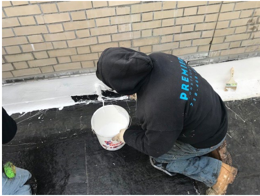
Figure 9: apply to prepped and primed substrate with roller.
