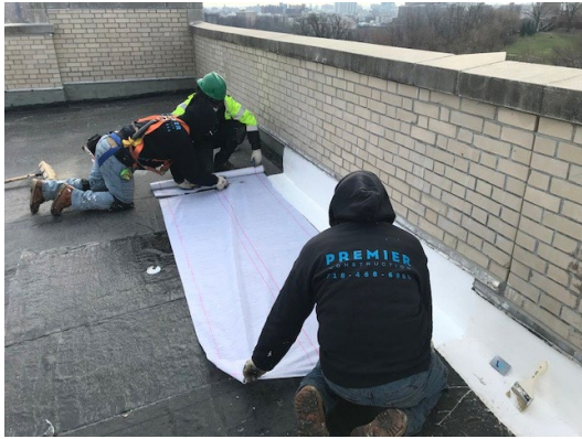
Figure 11: install fleece reinforcement.
