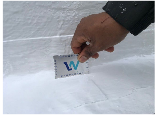
Figure 10: verify first resin application is 45 mils wet thickness (min)
