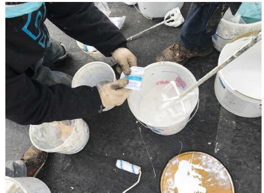
Figure 8: thoroughly mix and evenly disperse catalyst into resin.
