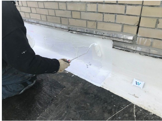
Figure 15: overlap 2-inches on existing PMMA as required.
