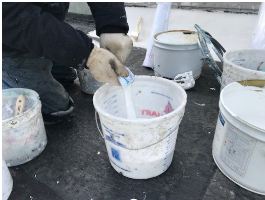
Figure 7: add PMMA catalyst as required to PMMA resin.
