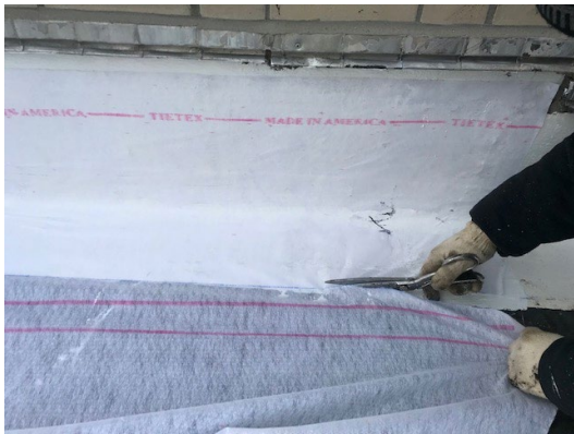
Figure 13: cut leading edge of fleece ¼-inch from edge of resin.
