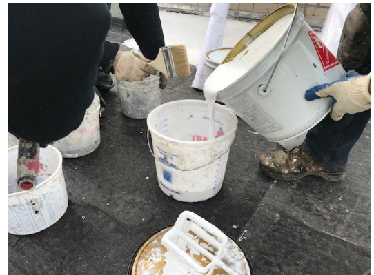
Figure 6: use and catalyze what is needed for the installation.
